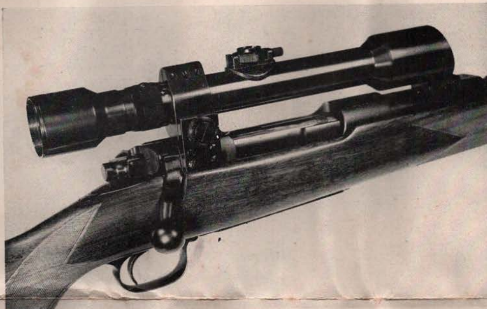
Stith Custom Mount, with windage adjustment shown here with Hensoldt 4X scope. Model 70 mount design is adaptable to other bolt action rifles.
