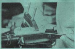
On the Krag, care should be taken so that shell will properly eject. Centerline of scope will have to be offset to left, approximately % inch, approximate location, so bottom of base mount is about 1/32 inch from top of magazine plate. Above illustration (left) shows drill jig in approximate position. Be sure stop pin rests on receiver bridge. Adjust spring catch so scope is held securely.
